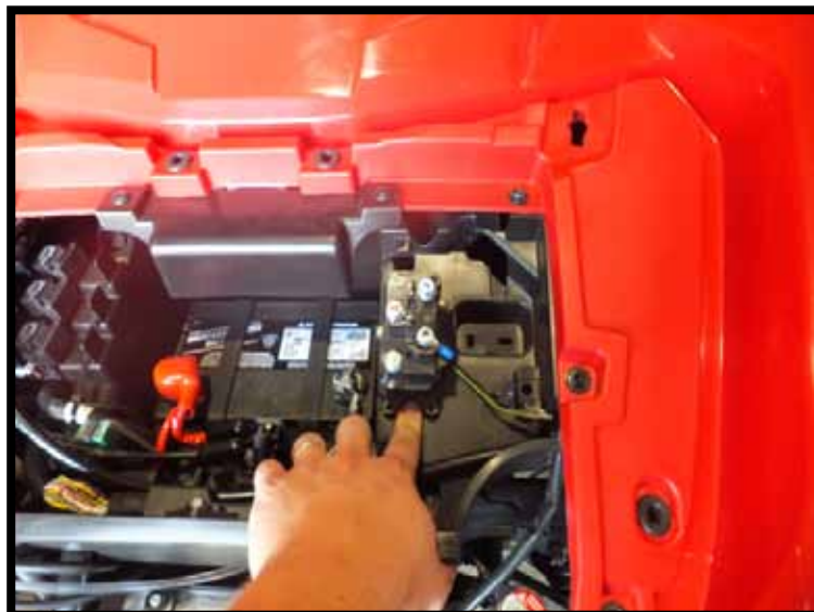
“Figure 8” Contactor Location
