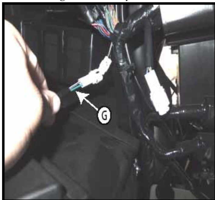
“Figure 11” Wire Location Under Passenger Side Fender
