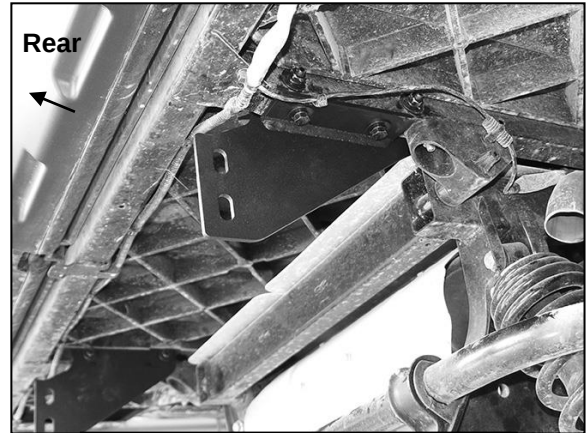
(Fig 9) Frame Brackets installed
