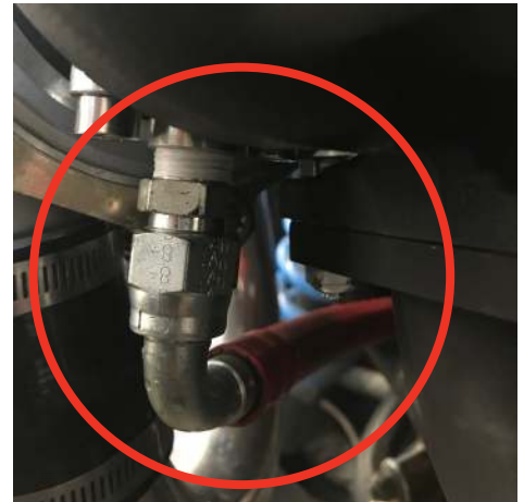
19. Install oil drain into the bottom of the turbo assembly.
